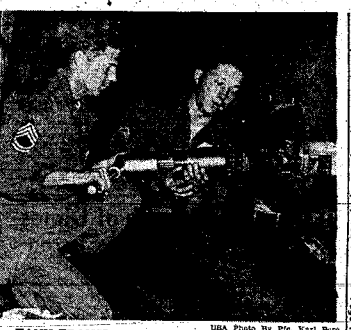
TANK TRANSPORTER REPAIRED BY CTC MEN - Sfc. H. Bates and Cpl. C. Riley at Work
