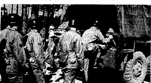
LEAVING FOR BIVOUAC AND TRAINING ARE THESE MEN OF THE IOCS
