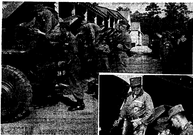
OPERATION ANTI-FREEZE . . . First Lt. Ernest G. King, center, with arms folded, motor officer of the 508th ARCT, supervises cold-weather preventive maintenance of heavy-duty trucks. At right, 508th personnel take hydrometer reading after pouring a 'shot. They are, left to right, Pvt. Cesario Ramirez, Sfc. James L. Russell, and WOJG Louis W. Strace.
